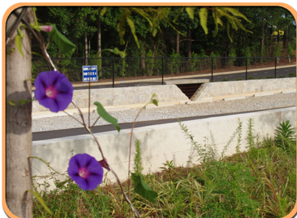
The lowest row of bioretention cells overflow directly into the gravel cellular infiltration basin, which also serves as parking. This pervious area helps filtrate and treat stormwater. This photo shows the distinct ponding line that has been carefully maintained in each cell.
