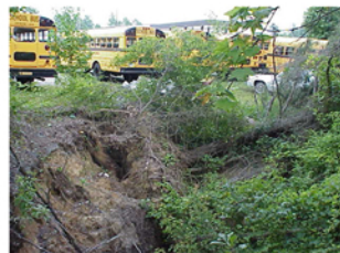
These views of the adjacent property to the west illustrate the level of erosion downstream from the new parking lot site.
