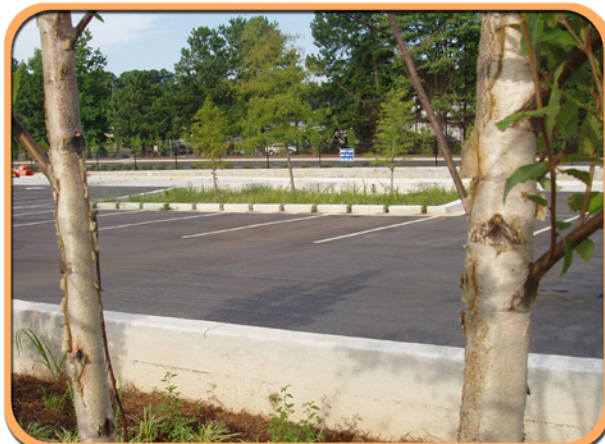
The bioretention cells are staggered throughout the parking lot. These cells are planted with material, such as River Birch (Beula nigra) and Bald Cypress (Taxodium disticum) which are well adapted to survive in xeric and mesic conditions. These cells also help cool the surface temperature of the parking lot, helping reduce the heat island effect.
