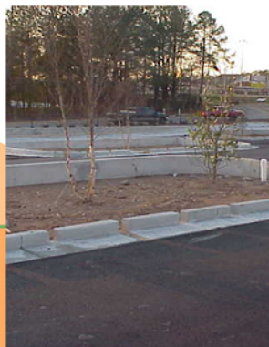
The top coat of asphalt and the plant material is placed.
