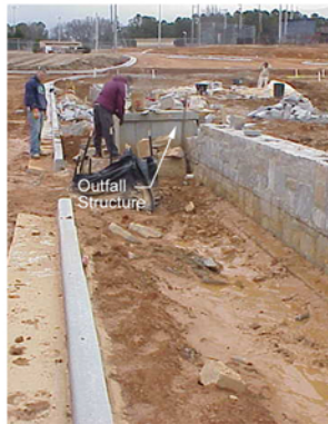
The outfall structure and the granite detention wall is constructed.
