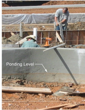
As work continues, the ponding levels of the bioretention cells are established.
