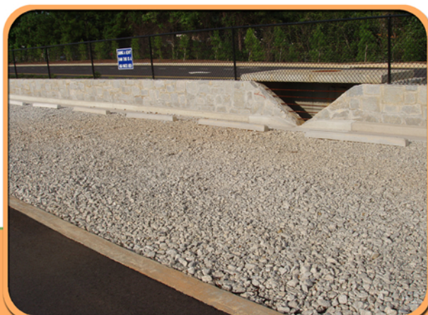
In severe rain events, water which is not infiltrated becomes detained against the granite wall and discharges through the "V" notch orifice.
