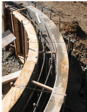
One of the bioretention cell walls is formed.
