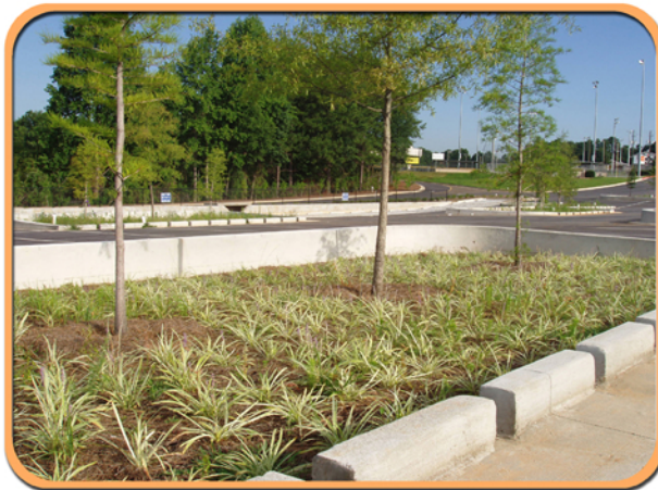
Rectangular concrete weir notches help control stormwater velocity entering the bioretention cells and also act as wheel stops. In large rain events, stormwater fills the cell to the ponding limit, then spills back out through the weirs, running down hill to either another bioretention cell or to the cellular infiltration parking and detention.
